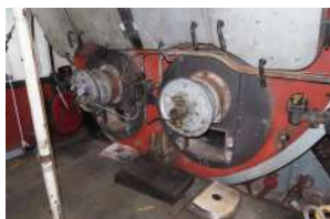
Wattle Engine room
